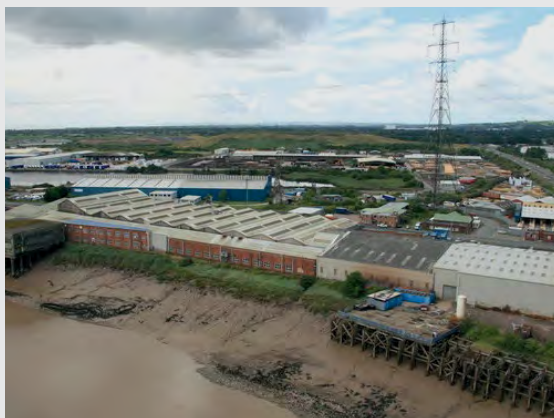
ABP South Wales buys new property at Newport to accommodate growth
